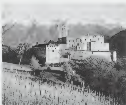
Coira Castle in the Venosta valley of the upper Adige River, in the Ötztal Alps, Italy
